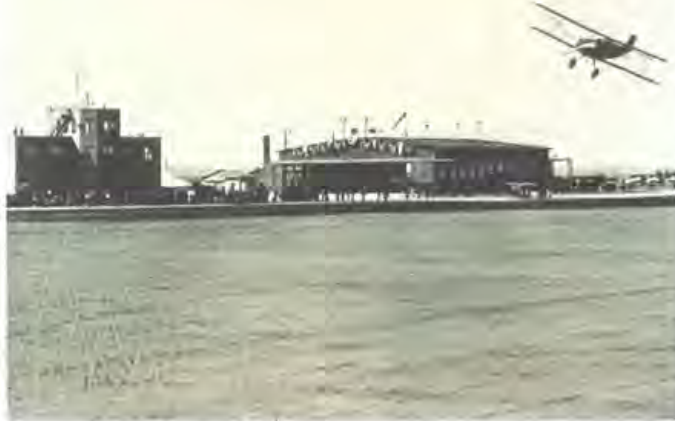
The Denver Municipal Airport opened for business in 1929 on "the Sand Hills site" east of Park Hill - considered by many to be too remote. It was renamed after Mayor Ben Stapleton in 1944.
