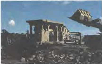
Recycling of Airfield Paving
